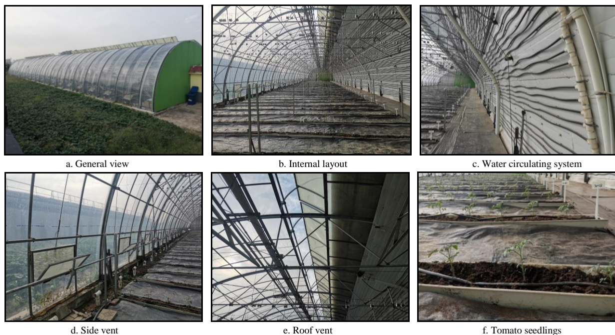
Figure 1 Examples of photographic views of sliding cover solar greenhouse and principal components
