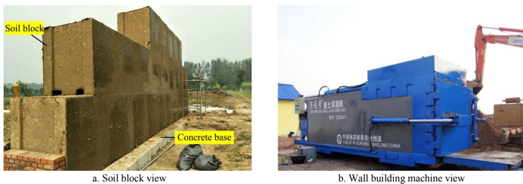
Figure 3 Soil block making and wall assembly process
